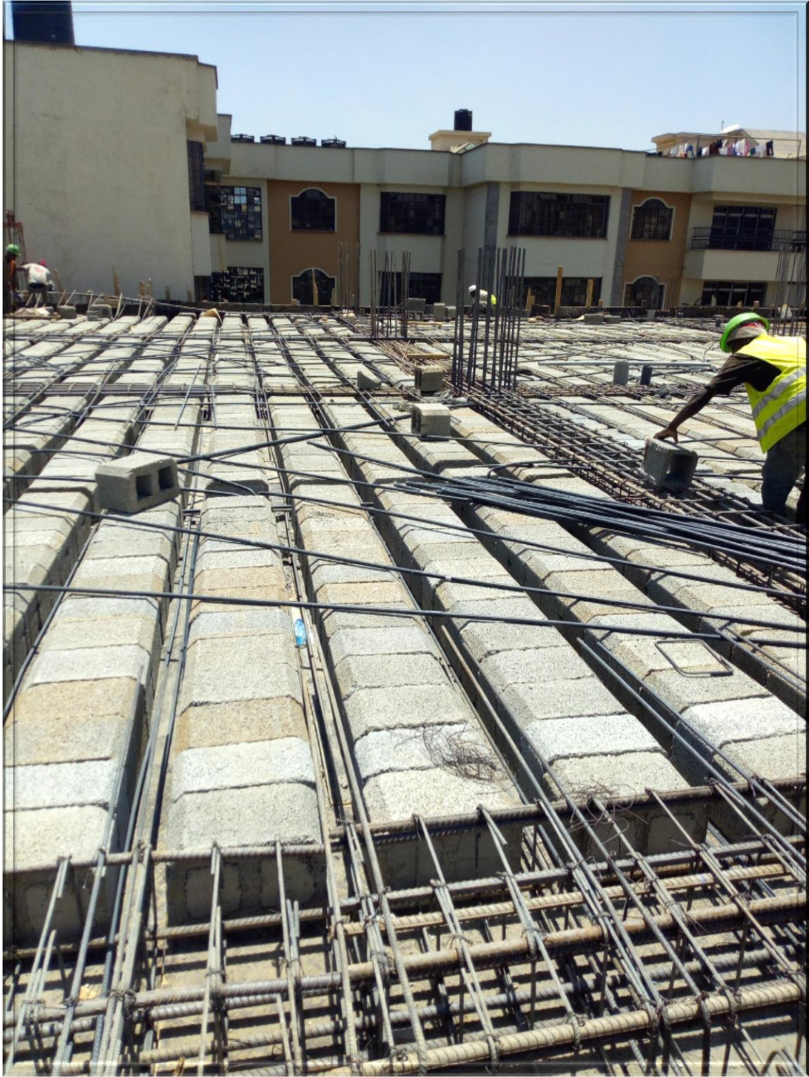
Fig. 03. Construction works going on as below
