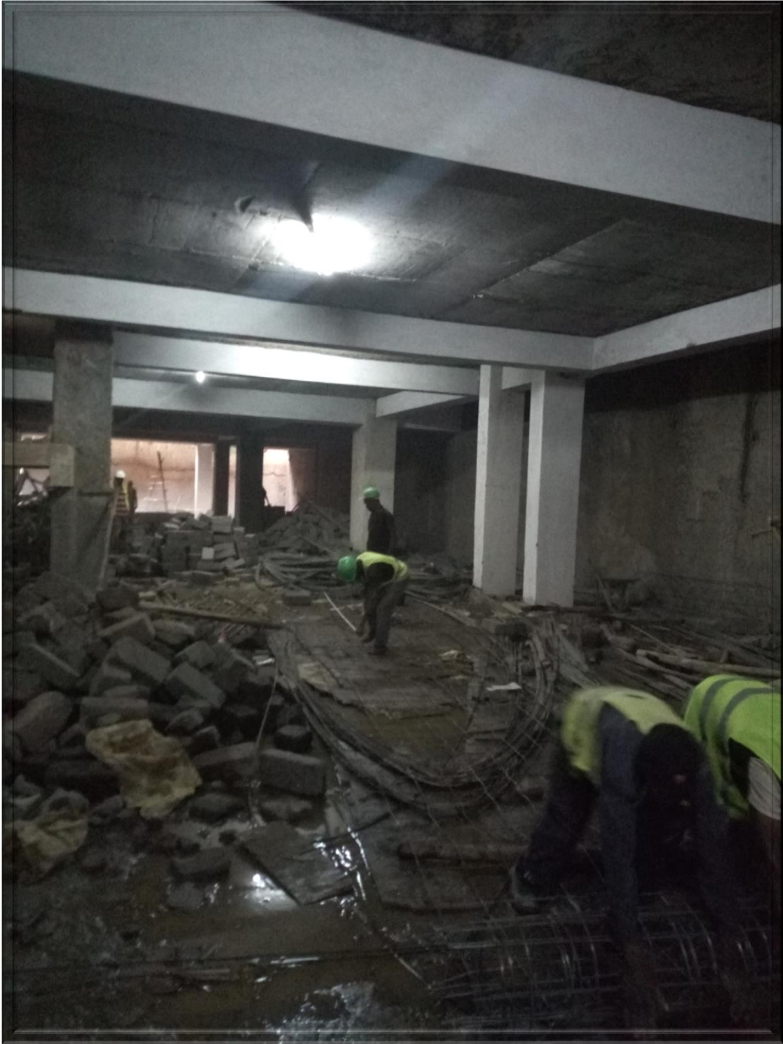
Fig. O2. Plaster works progressing on as below
