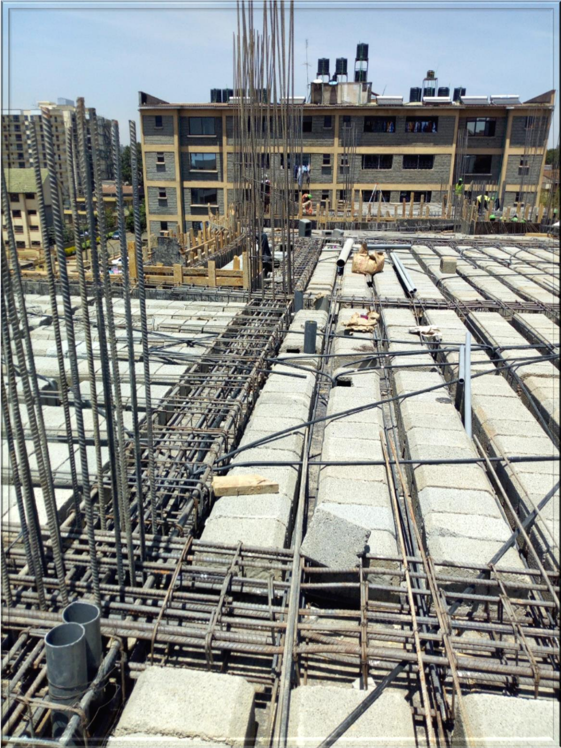
Fig. 06. Concreting works progressing on as below
