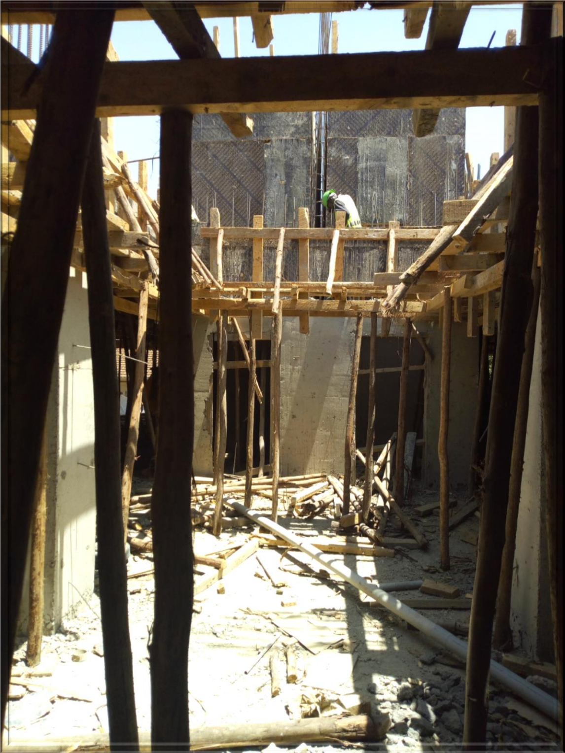
Fig. 04. Lift shaft construction in progress
